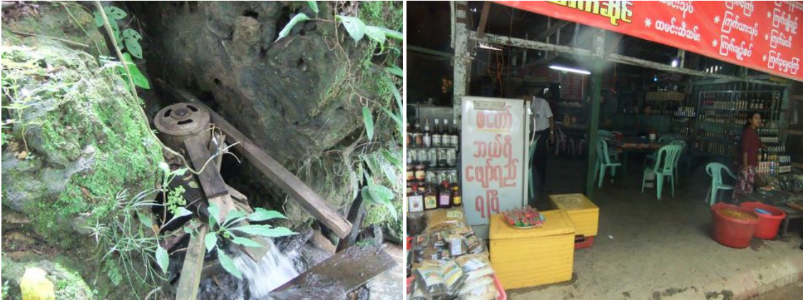
Mini-hydro Turbine in Waterfall Powering Restaurant w/ Refrigerator, Lights & TV
