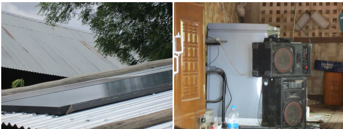
Solar panel used to power store refrigerator, lights and sound system in Monywa
